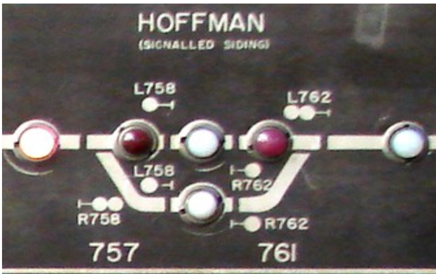
Portion of a former Seaboard Air Line CTC panel, Hoffman, NC. This panel is now located at the NC Transportation Museum, Spencer, NC.
